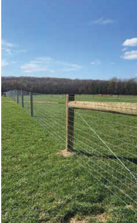
These three images show 2,000+ feet of Bull Barn 13/48/4 fence installed by Ridgeline Fencing LLC. The project involved tying into old fence from a previous contractor, dividing pastures, and adding several new paddocks.
