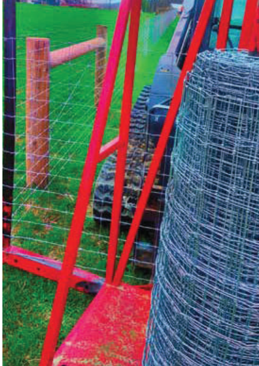
These three images show 2,000+ feet of Bull Barn 13/48/4 fence installed by Ridgeline Fencing LLC. The project involved tying into old fence from a previous contractor, dividing pastures, and adding several new paddocks.
